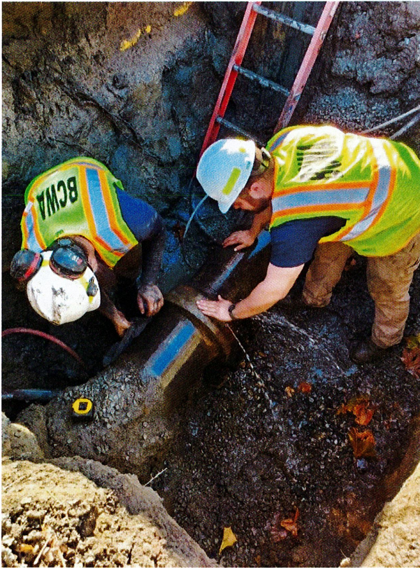
Figure 3a. Cast Iron Bell Joint Failure
